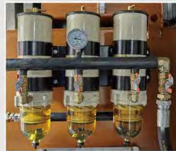
Three layers of water-fuel separation device
